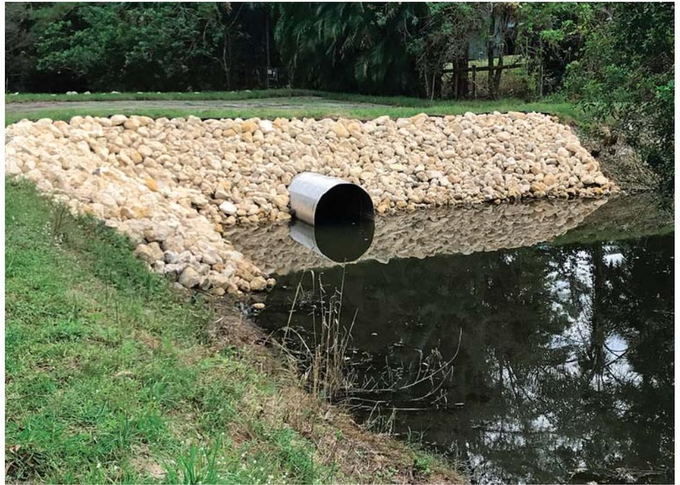
Culvert installation across Canal 8 just east of Canal 10 allows for additional access to the canal system - it included the installation of approximately 60 feet of 48-inch diameter pipe, fill material, rip rap, and sod
